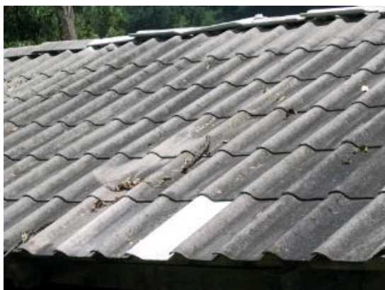
Figure 3.4 Concrete tiled roof
